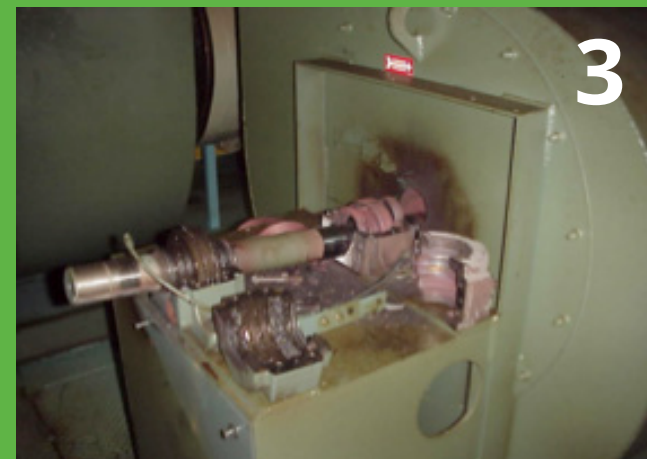
BEARING LUBRICATION
