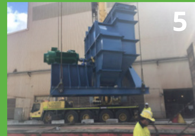
FAN DELIVERY & INSTALLATION
